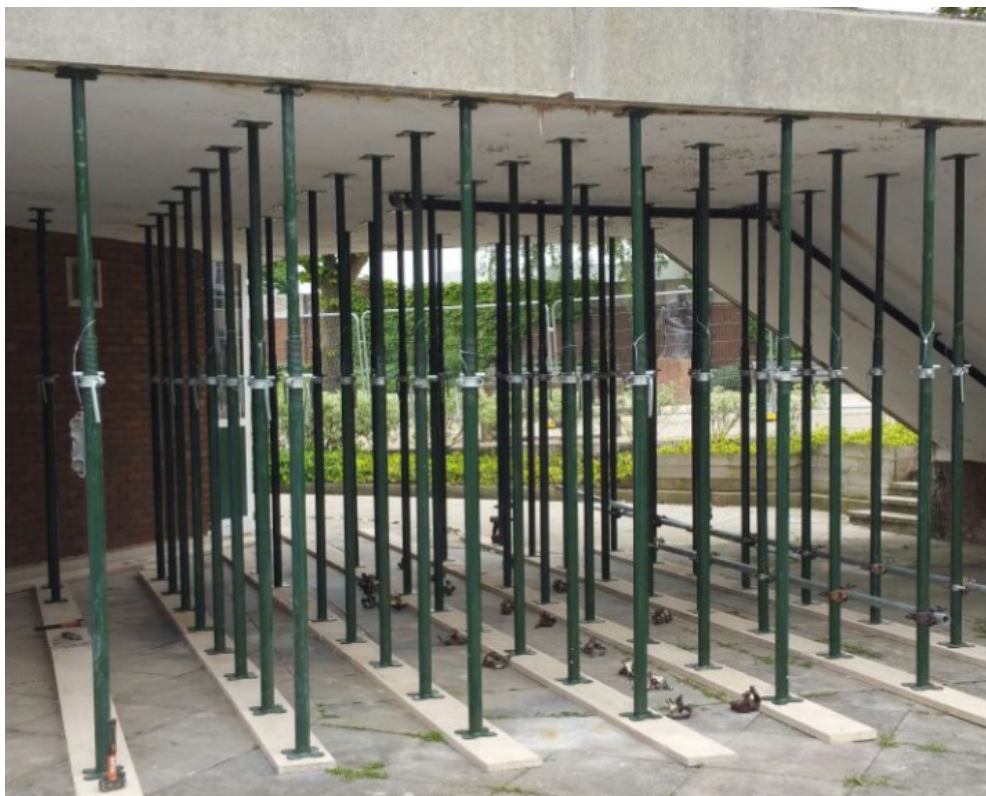
Vertical & Plumb Acrow props (in the process of being braced)
