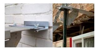
The main cause of collapse is overloading equipment due to the working load being variable. When using the last 100mm of the tongue, it bends from a load of 50kg and will only support the front edge of the masonry which causes further instability.
