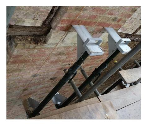
With over 30 years experience within the construction industry I have yet to see Strongboy's being used correctly which I believe to be due to a severe lack of correct guidance. Yes a Strongboy supports masonry but not safely, it is more luck than any structural engineer's calculations or judgement.
