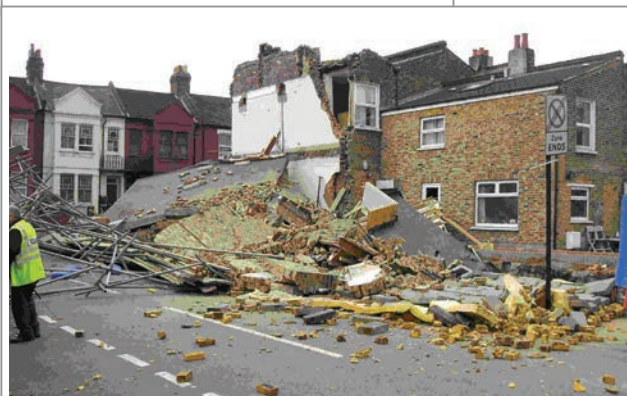
Complete collapse of a refurbishment, which included the construction of a new basement.
