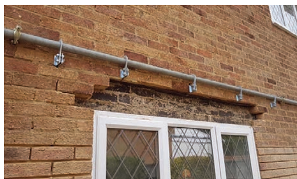
Figure 3 Brick Brace Safety Tool and Safety System
