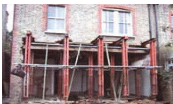
Figure 2 A strong, reliable system of needling
